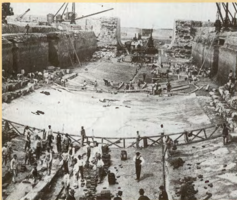
Excavation of Port of Buenos Aires, Argentina Relying on foreign capital and engineering, the government of Argentina improved the port to facilitate the nation's rapidly expanding export economy. (Courtesy, Hack Hoffenburg, South American Resources)
