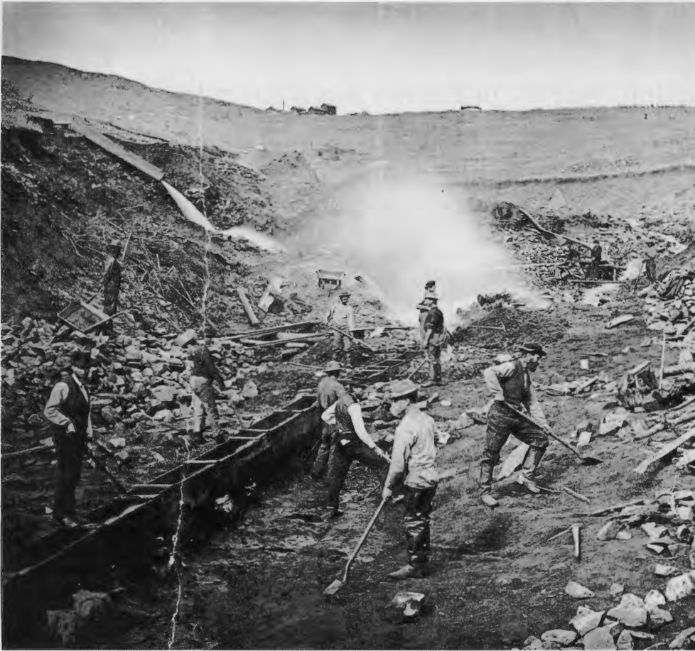
The Introduction of New Technologies Changes the Mining Industry Powerful hydraulic technologies were introduced in western mining sites in the United States. This early photo shows how high-power water jets could transform the natural environment. (Colorado Historical Society)
