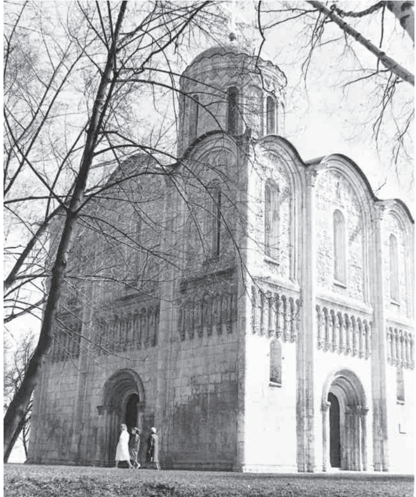
Cathedral of Saint Dmitry in Vladimir Built between 1193 and 1197, this Russian Orthodox cathedral shows Byzantine influence. The three-arch façade, small dome, and symmetrical Greek Cross floor plan strongly resemble features of the Byzantine church shown on page 256.
